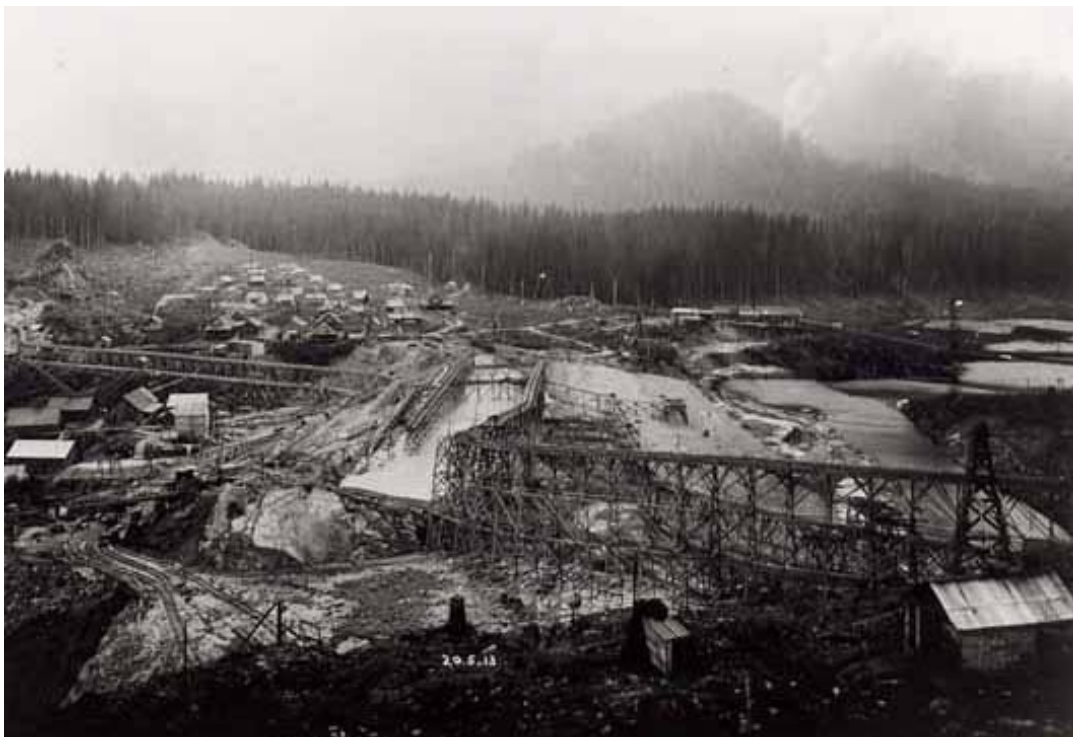
Photograph 1. Final phase of the Coquitlam Dam - 1913. Photograph from Koop, 2001.
