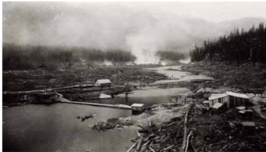
Forest clearing and pile burning operations for 70 foot flooding margin at the south end of Coquitlam Lake, around 1911. Source: B.C. Hydro archives.
