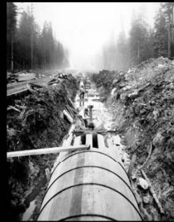
Wooden Water Main - circa 1910
