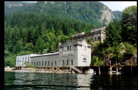
Power Station at Indian Arm
